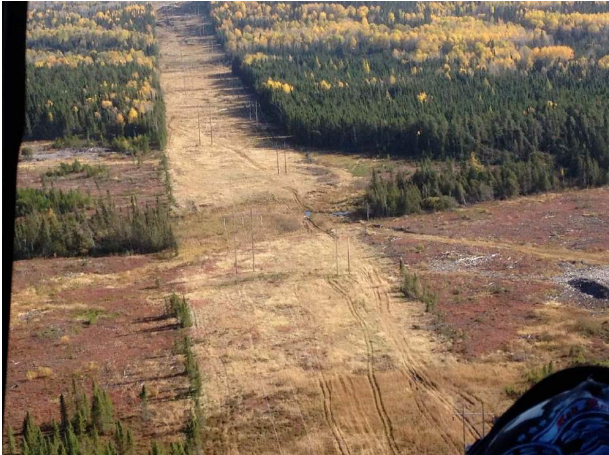
Figure 3.12-2: Power Line Infrastructure
